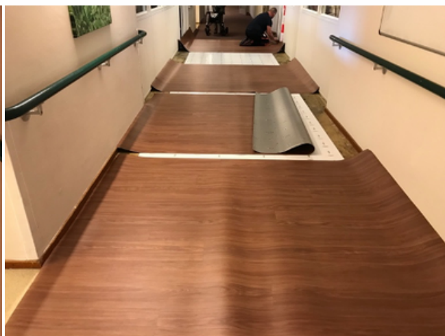
Image 4. Placing floor over sensor foil.
